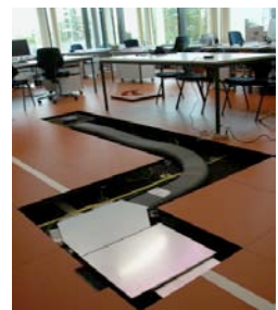
LowEx Technology: decentralized ventilation system with exhaust integrated into ceiling panels and controlled for optimized removal by CO 2 sensors (left), and subsequent optimized air intake system coming directly through the facade in compact systems integrated into the floor (right).
